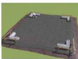
2 Place gas membrane/dpm. Turn perimeter down and allow 1m overlap. Lay 3-8mm stone blinding up to 50mm deep. Set out corners.
