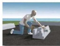
3 Continue placement of ring beam profiles. Trim profiles as necessary to achieve a tight fit. Join profiles with galvanised steel combs.
