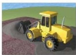
1 Strip site and lay compacted hardcore compacted in 50mm layers (18-35 mm hardcore). Incorporate Radon sump and pipework
