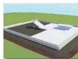
4 Place first 2 layers of floor insulation sheets over the remaining foundation. Overlap sheets to achieve continuity of insulation.
