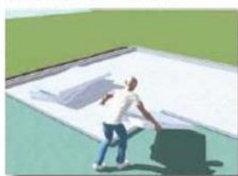
5 Install the final layer of insulation. Secure with EPS nails.
